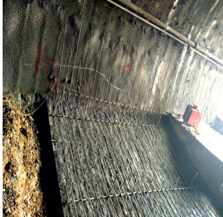
Inverted Arch Shotcrete
