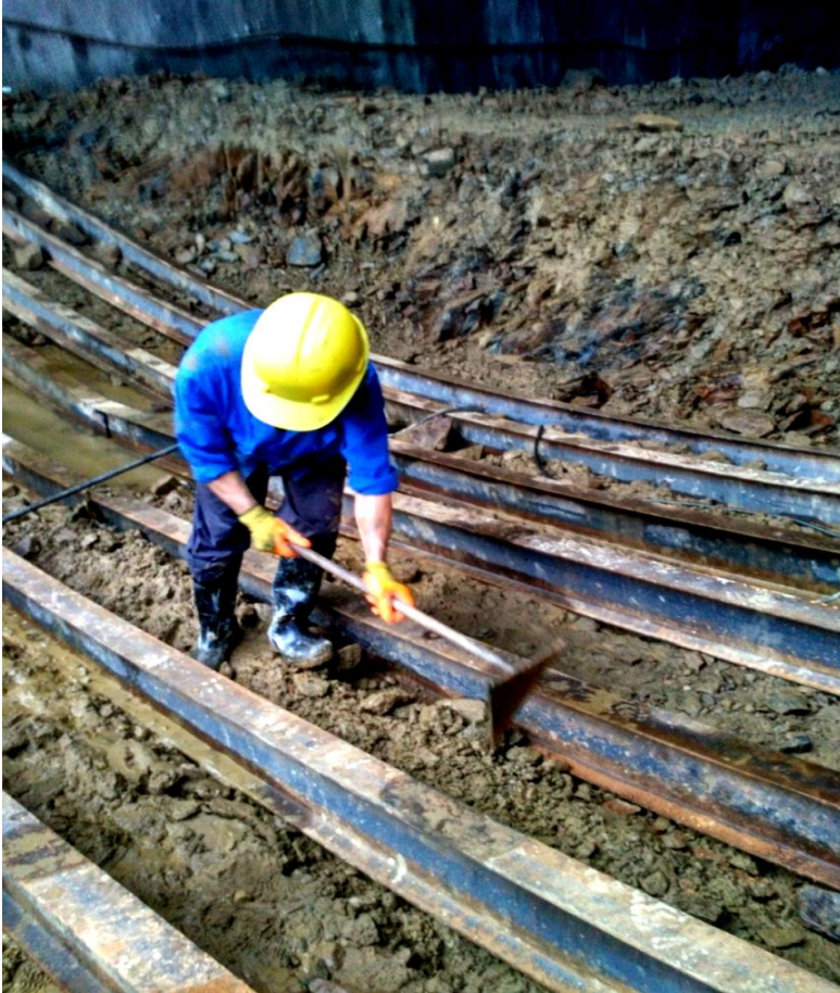
Inverted Arch Steel rib
